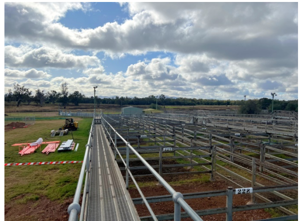
Works commenced on the major upgrade of the Gunnedah Regional Saleyards.
