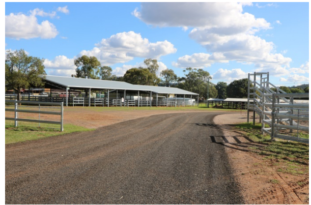
Upgrades were undertaken to the roads within the Showground Precinct
