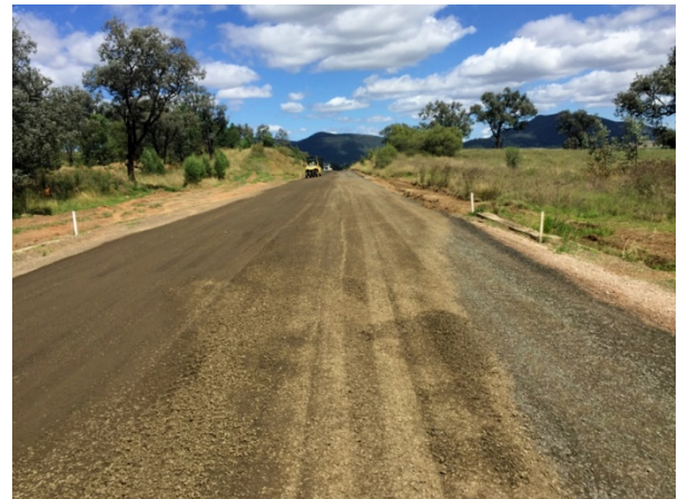
Sealing of Kelvin Road well under way
