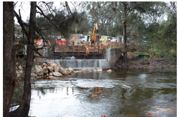
Orange Grove Bridge under construction
