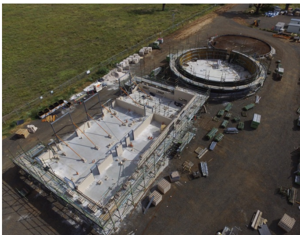
Water Treatment Plant under construction
