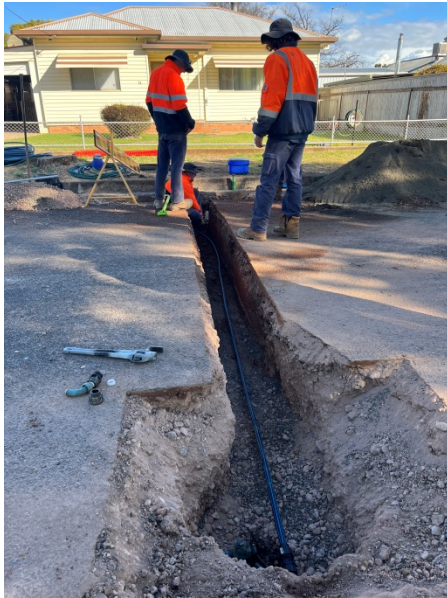
Kilcoy Street mains replacement
