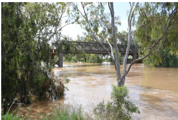
Cohens Bridge during the flood event in November 2021
