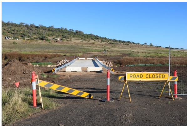
Bridge at Maitland Street, Breeza under construction
