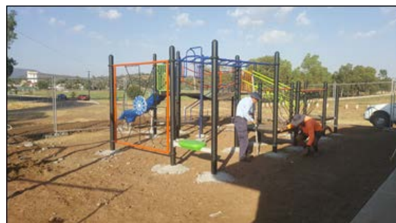
Installation of playground equipment at Donnelly Fields.
