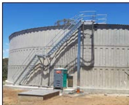
Ladder installed at the newly constructed Apex Reservoir.
