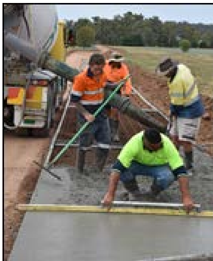
Council staff working on the Wandobah Road cycleway.
