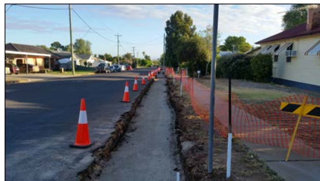
Bridge Street kerb and gutter construction works.
