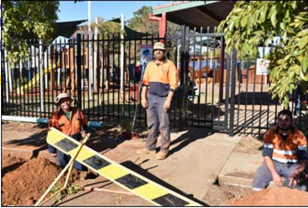
Council staff working on the sewer main replacement in Elgin Street.
