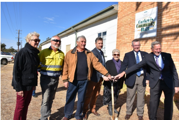
Councillor Gae Swain, TCM Civil Pty Ltd Director Colin Kiely, Councillor Rob Hooke, Mayor Jamie Chaffey, Councillor Colleen Fuller, Federal Member for Parkes Mark Coulton and Councillor Owen Hasler at the official sod turning of soil for the construction of the Curlewis Pipeline in July 2018.
