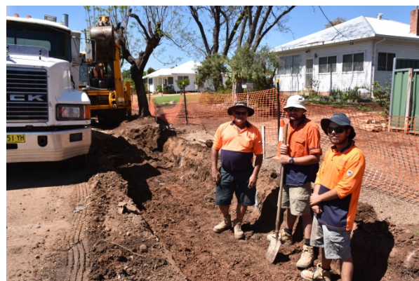
Council staff completing kerb and gutter works in Bloomfield Street.
