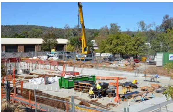
The Gunnedah Memorial Pool Complex Upgrade construction well underway.
