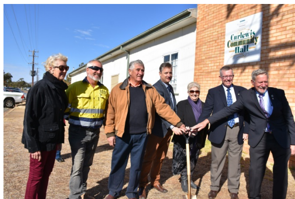
Member for Parkes, Mark Caulton, and Member for Tamworth, Kevin Anderson, with Councillors at the official sod turning for the construction of the Curlewis Pipeline.
