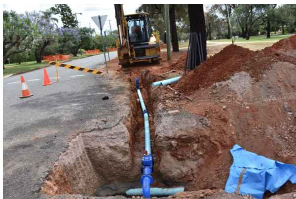
Stock Road main replacement.
