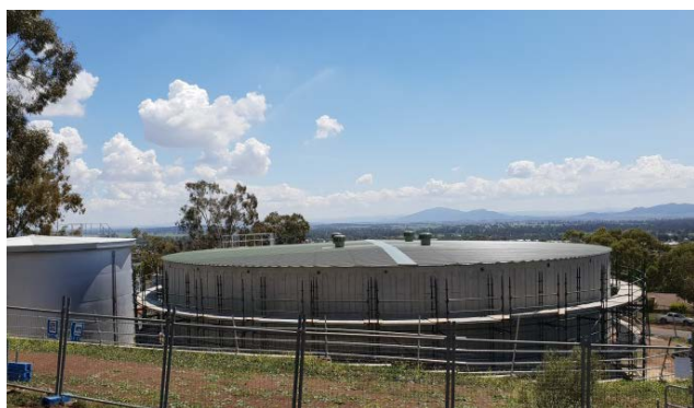
Apex Road Reservoir under construction.
