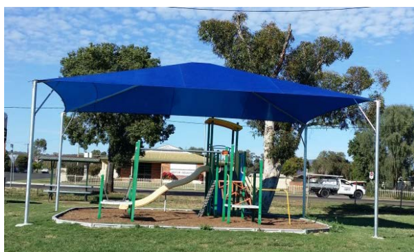
Shade sail installed at Kitchener Park.
