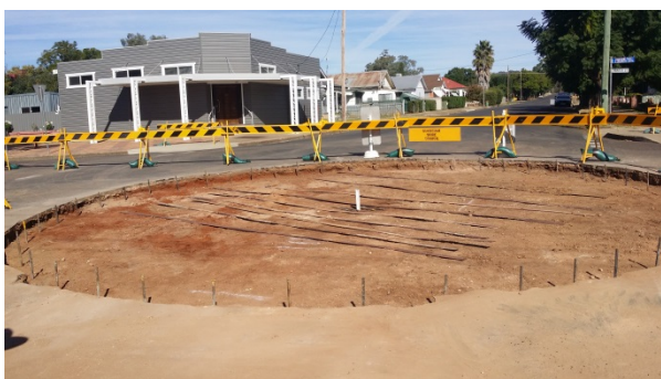
Construction of roundabout at Hunter Street/Rodney Street/Marquis Street intersection.
