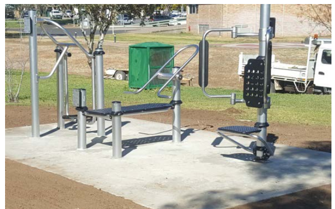
Gym equipment installed at Lions Park.
