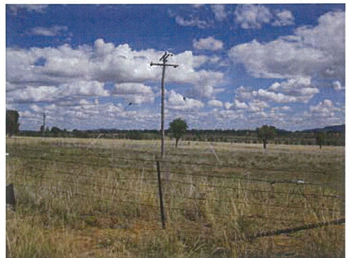
Existing power in south eastern corner of the chicken paddock
