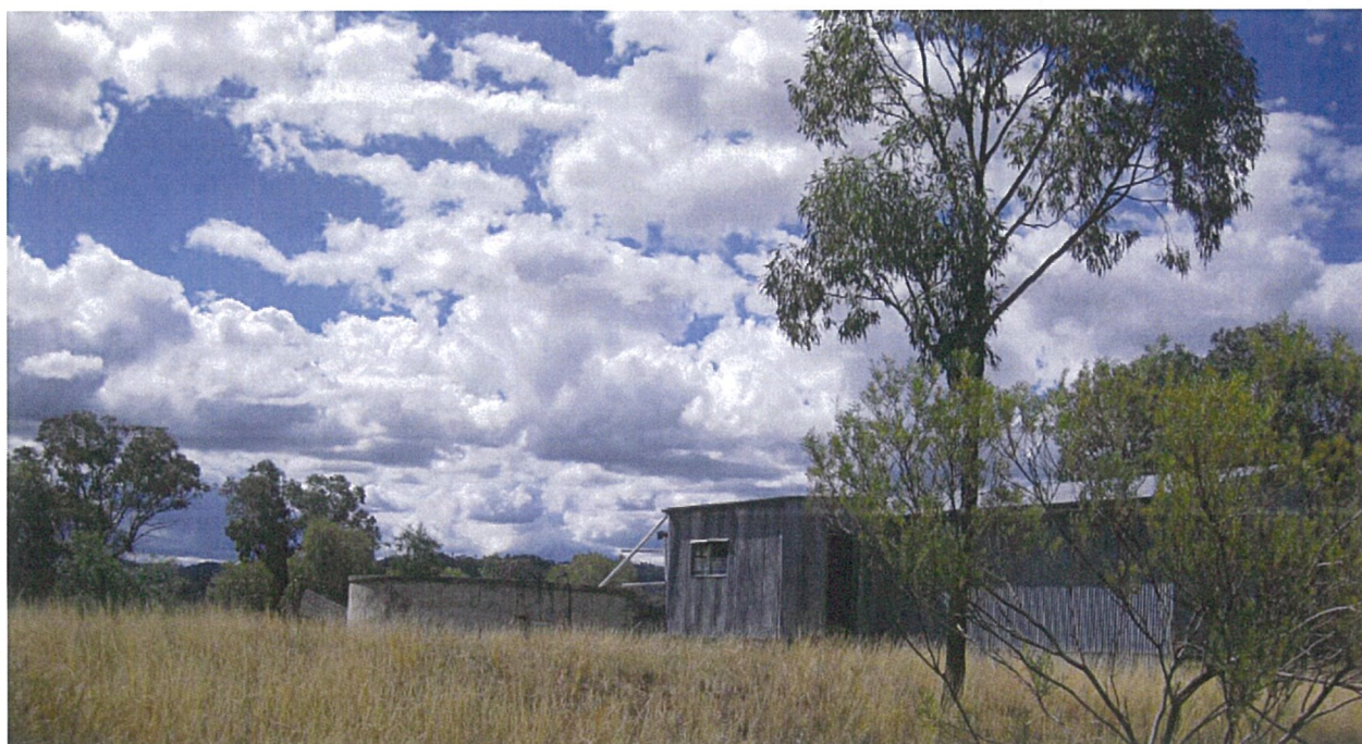
Figure 5: Existing Concrete Storage Tank which will supply Chook Sheds.
