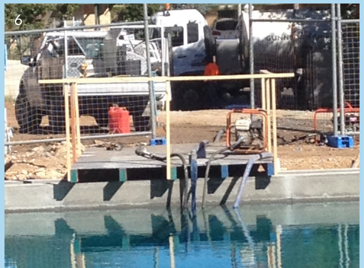
Photos 1 - 4: Time lapse images of pool being filled. Images taken at 7.00am, 11.00am, 4.00pm and when full. Photo 5: Pool full of water and not a leak! Photo 6: Pumping out the water for reuse.
