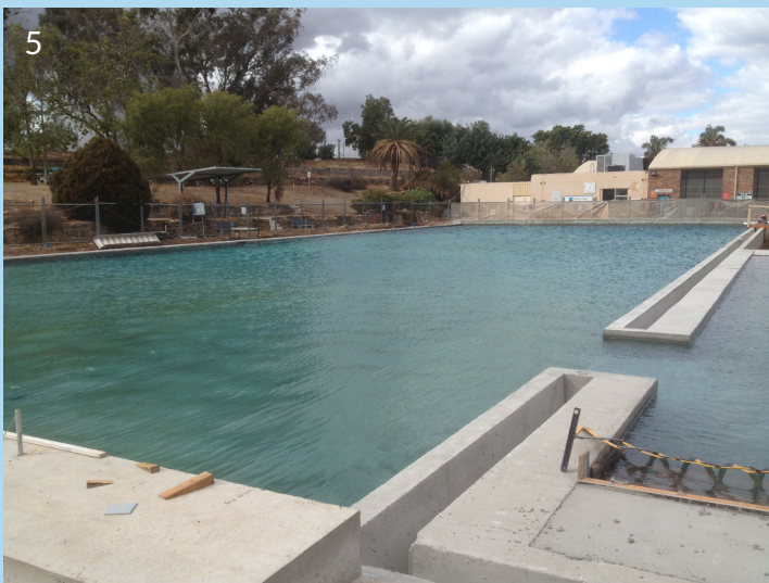
Photos 1 - 4: Time lapse images of pool being filled. Images taken at 7.00am, 11.00am, 4.00pm and when full. Photo 5: Pool full of water and not a leak! Photo 6: Pumping out the water for reuse.
