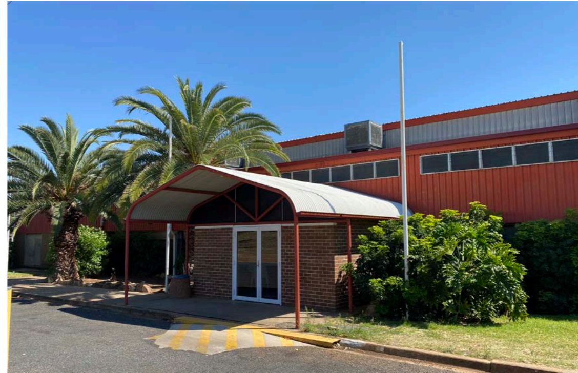
4. The Lyle Griffiths Gymnasium is one of the largest, and most utilised spaces
