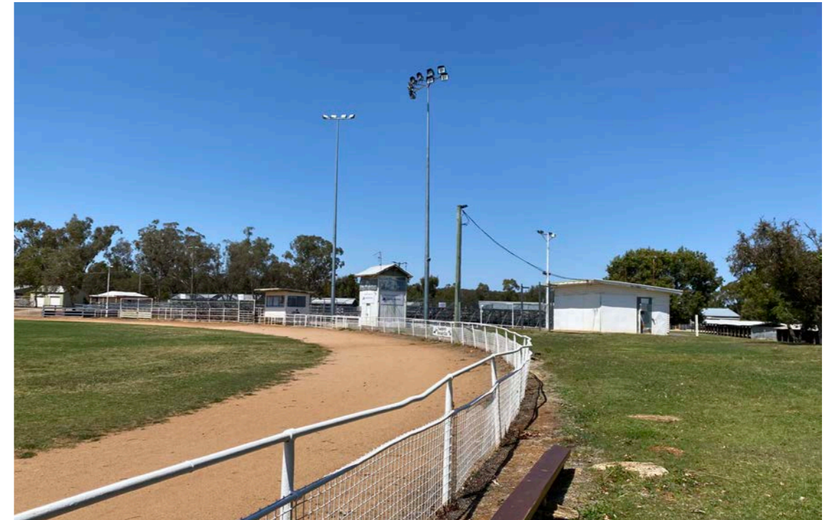
2. Cluster of buildings adjacent to the central arena, facing the softfall arena
