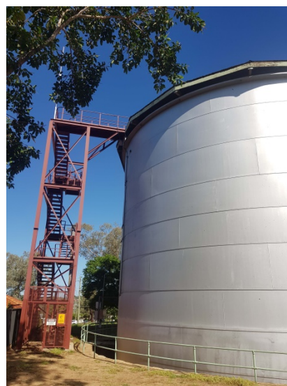
Works being completed on the South Street Reservoir.
