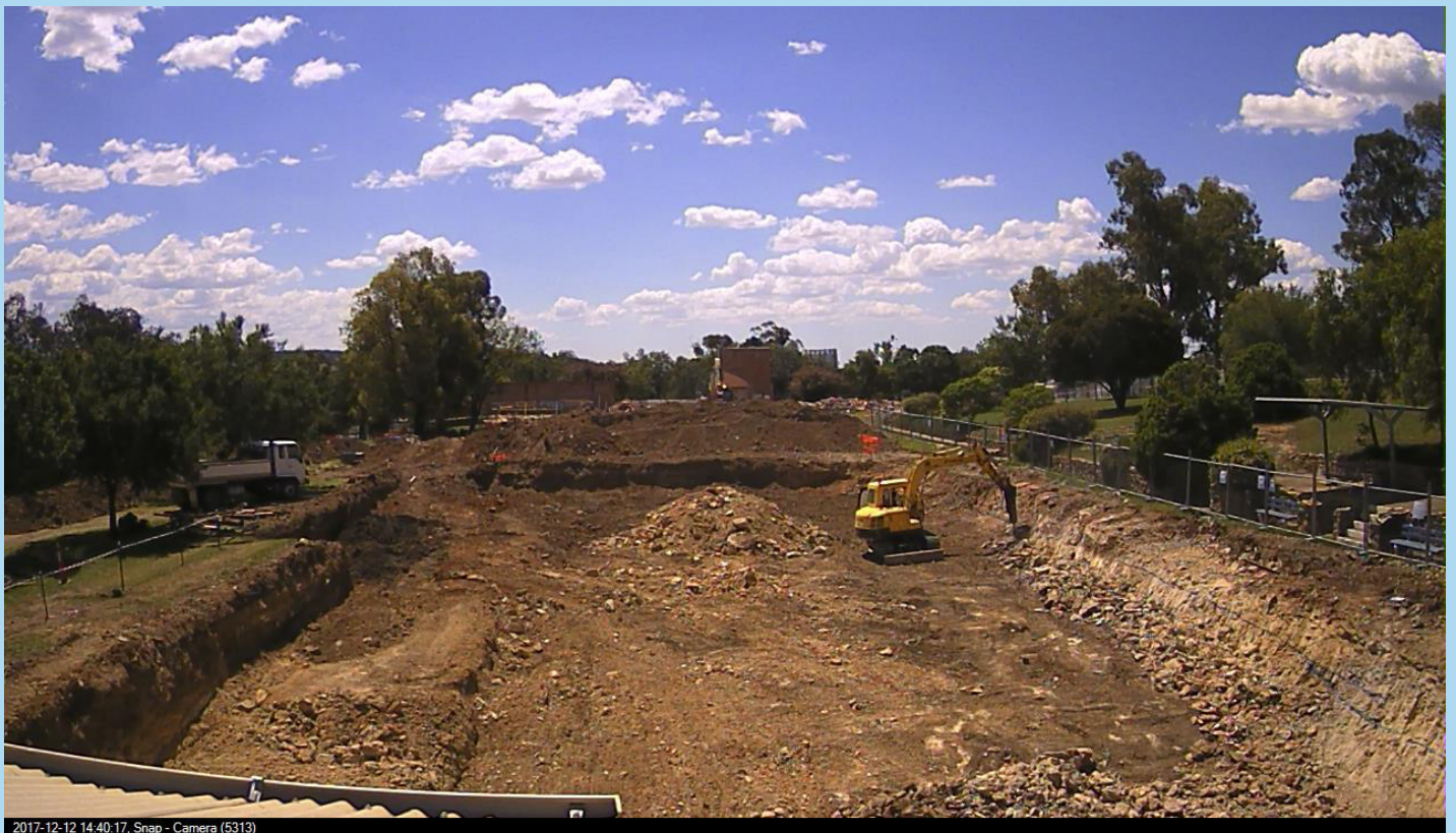
Photo: Demolition work on the Gunnedah Memorial Pool Complex as captured by the digital time-lapse camera.
