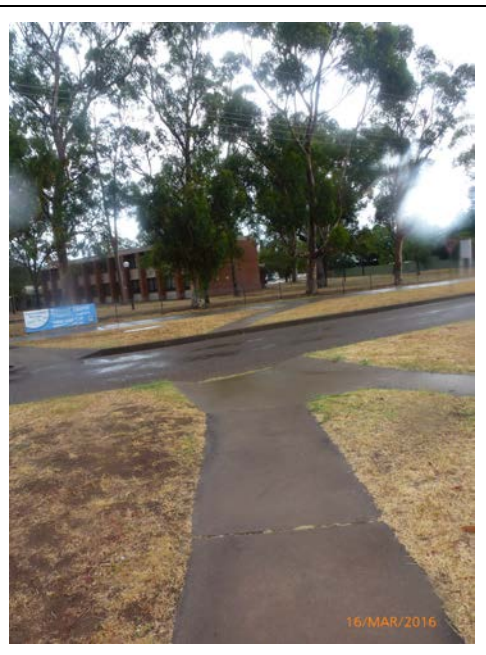
Plate 19 - Commencement of the shared path at the Hunter Street intersection
