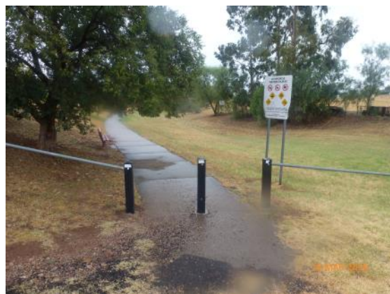
Plate 7 - Commencement of shared path at Lincoln Street
