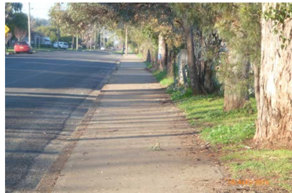
Plate 10 - Links Road shared path
