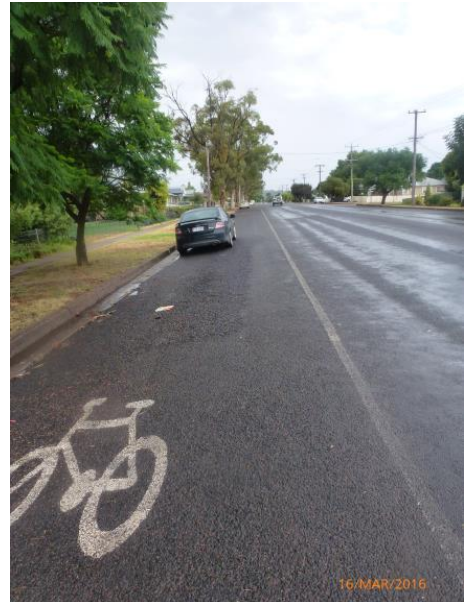
Plate 16 - On-road cycleway between George Street and Wandobah Road
