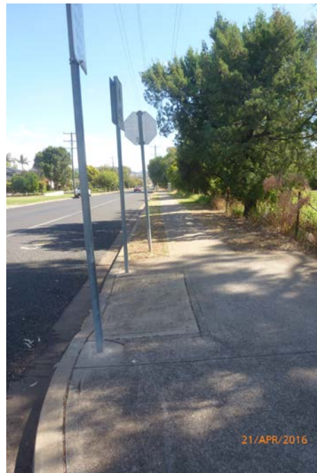
Plate 12 - On-road cycleway looking west from Links Road
