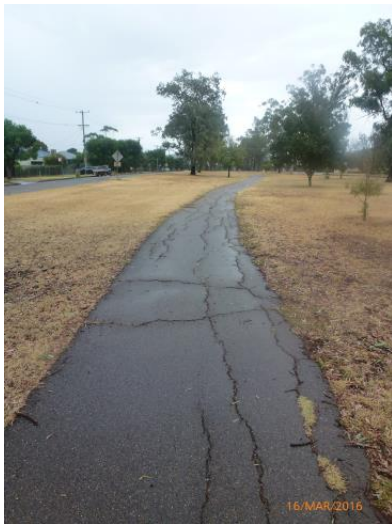
Plate 3 - Bitumen section of Stock Road shared path
