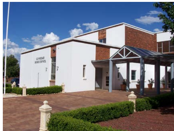
Council Administration Building,
