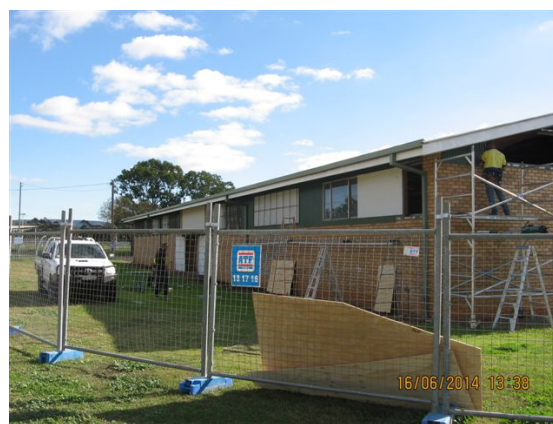
Asbestos removal at Griffiths Pavilion
