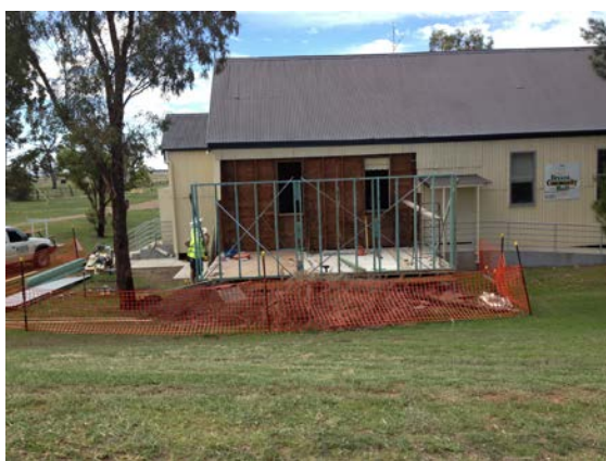
Construction of the new amenities addition to the Breeza Hall
