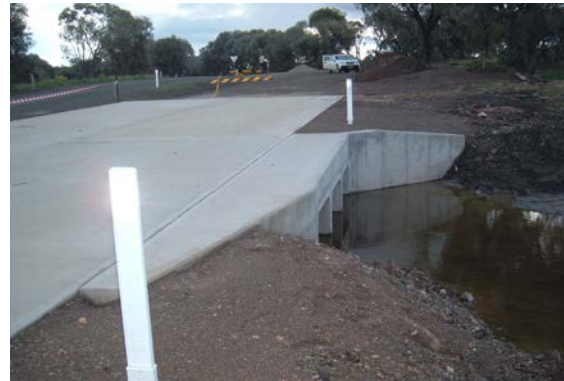
New culvert MR357 under and over
