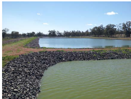
Curlewis Sewerage Treatment Plant
