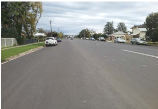
Bloomfield Street Upgrade – three blocks now complete
