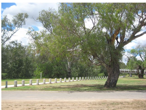
Installation of bollards at the Riverine area
