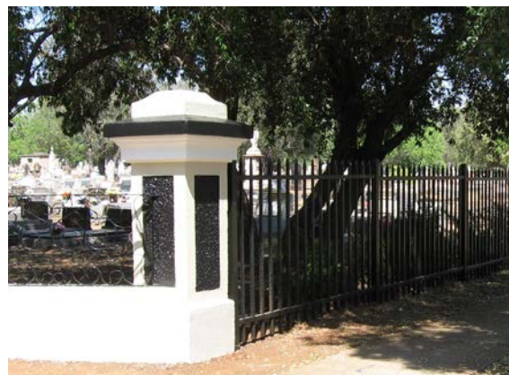
Hunter Street Cemetery new fencing and gates
