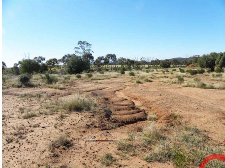
ERODED SOIL ABOVE THE CONSTRUCTED CHANNEL
